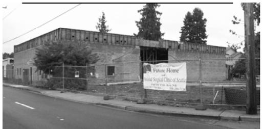
Construction is progressing well at this point. The inside of the current building has been completely demolished and the foundation for the new addition (on the South side of the existing building) has been poured. Framing of the interior walls in the existing structure is almost complete and we will begin framing the new addition in the near future (pending weather conditions). - Allen Johnson
