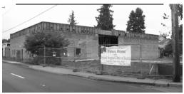
Construction is progressing well at this point. The inside of the current building has been completely demolished and the foundation for the new addition (on the South side of the existing building) has been poured. Framing of the interior walls in the existing structure is almost complete and we will begin framing the new addition in the near future (pending weather conditions). - Allen Johnson
